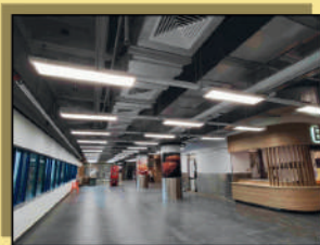
Renovation work of Building Services System (Canteen in City University of Hong Kong)
