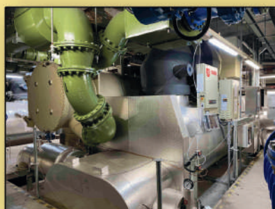
Replacement of 6800 Tons Chiller Plant System (Tuen Mun Hospital)
