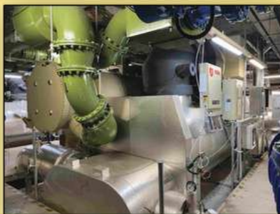
Replacement of 6800 Tons Chiller Plant System (Tuen Mun Hospital)
