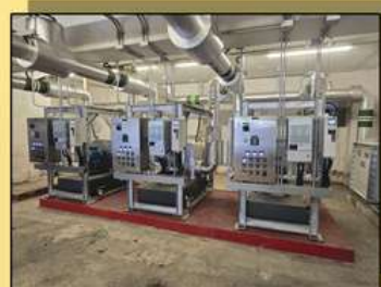
Multi-trade Integrated Mechanical Electrical and Plumbing (MiMEP) & Building Information Modeling (BIM) (Wang Cheong Building)
